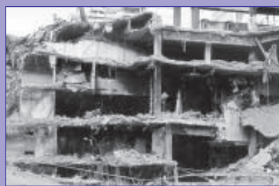
The World Trade Center recovery project: Demolition and stabilization on building 5
