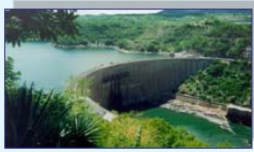
Hydroelectric Power Plant
