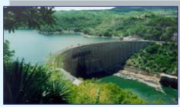
Hydroelectric Power Plant
