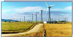
Wind Power Plant
