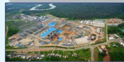
OC & CC Power Plant
