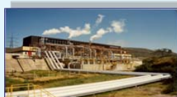
Geothermal Power Plant
