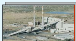
Coal fired Power Plant
