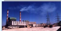
Oil fired Power Plant
