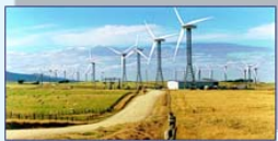
Wind Power Plant
