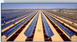
Solar Power Plant
